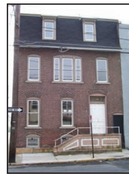
Chew Street Property Renovation Allentown PA
